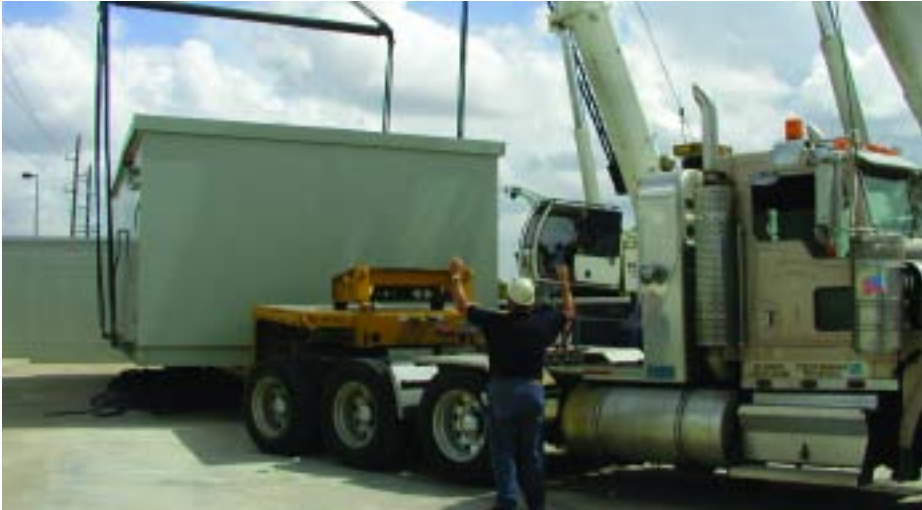
New cooling equipment is lifted into place. Photograph: Greg Mooney
